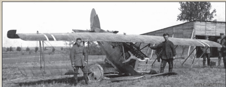
This crashed late production Pfalz D.XII is purportedly another from Jasta 49 but features numerous anomalies. The horizontal tailplane appears to have dark cordwise stripes and possibly a paler spanwise band under that which wraps around to the underside light blue. Additionally the wheels have not been painted a dark colour as per (B) and there is no cross on the rudder. Note how the right elevator has almost completely broken off in the crash and is hanging by its inner hinge point.
