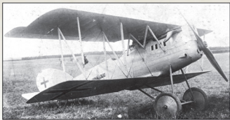
This crashed late production Pfalz D.XII is purportedly another from Jasta 49 but features numerous anomalies. The horizontal tailplane appears to have dark cordwise stripes and possibly a paler spanwise band under that which wraps around to the underside light blue. Additionally the wheels have not been painted a dark colour as per (B) and there is no cross on the rudder. Note how the right elevator has almost completely broken off in the crash and is hanging by its inner hinge point.
